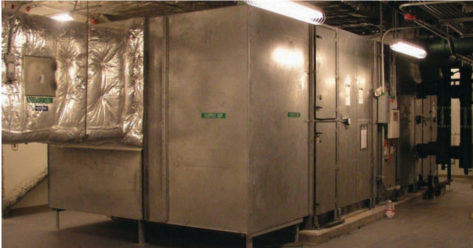
Cleveland Clinic Florida is equipped with Trane Climate Changer™ air handlers for efficient, quiet air distribution throughout the hospital and clinic.
