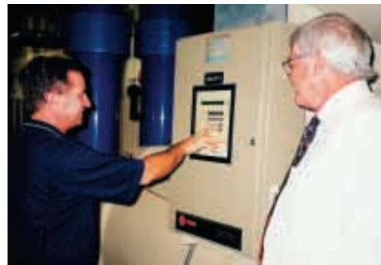
Chiller control system features Trane's Adaptive Control™, allowing the chiller to stay on line under adverse operating conditions.
