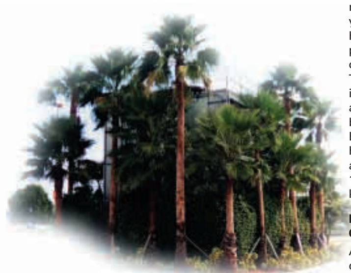
Cooling towers in the parking area are screened with palms to fit in with the tropical landscape at the stadium site.
